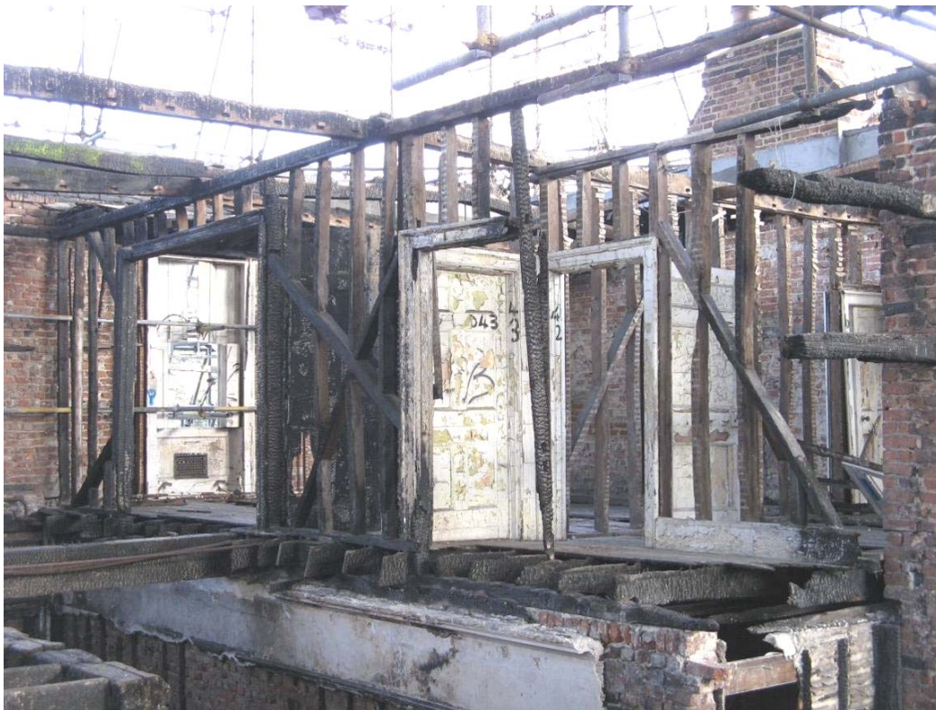
Figure 32: F1 internal partitions
