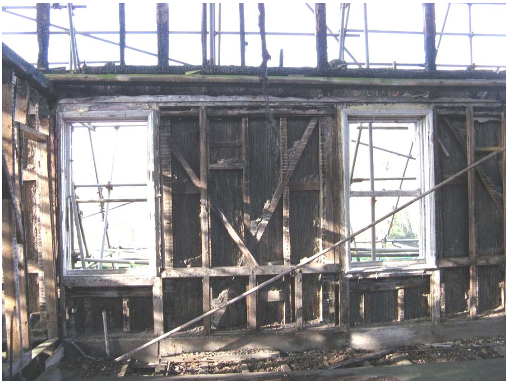
Figure 34: F14, undamaged timber framing
