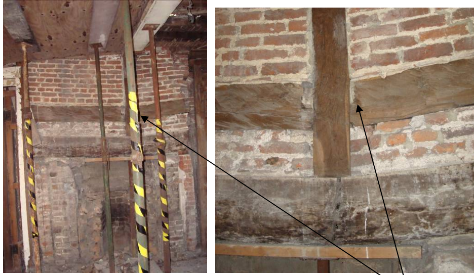
Figure 5: Cross-wing - ground floor chimneystack and detail of empty mortice for original floor structure
