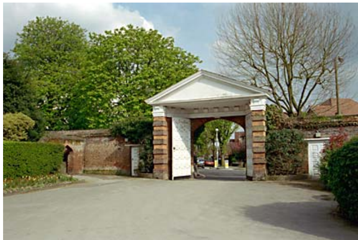
Figure 20: Entrance gate, inner face
