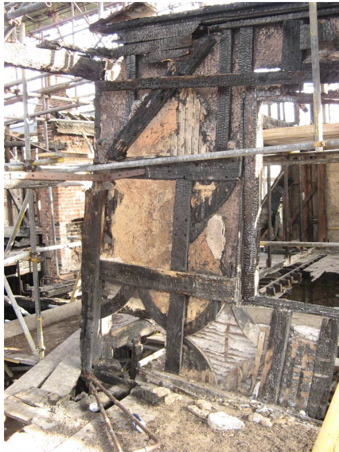
Figure 25: F12 cross-wing, remains of framing
