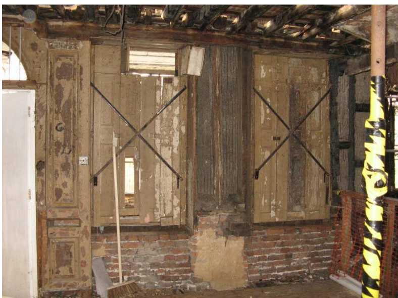
Figure 30: G4 18 th century joinery in situ
