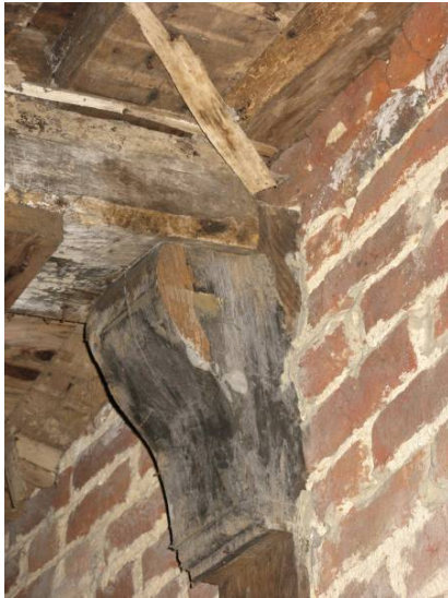
Figure 9: Inserted scrolled bracket carrying cross-wing floor
