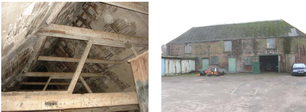
Figure 36: The stables, roof and north elevation
